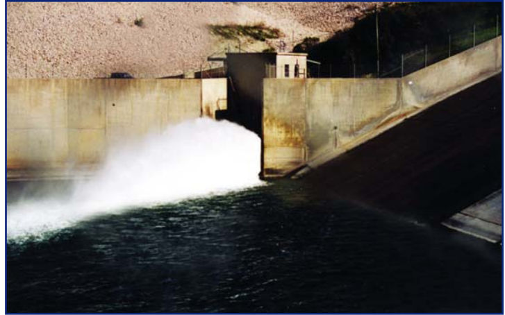
Free discharging fixed cone valve
