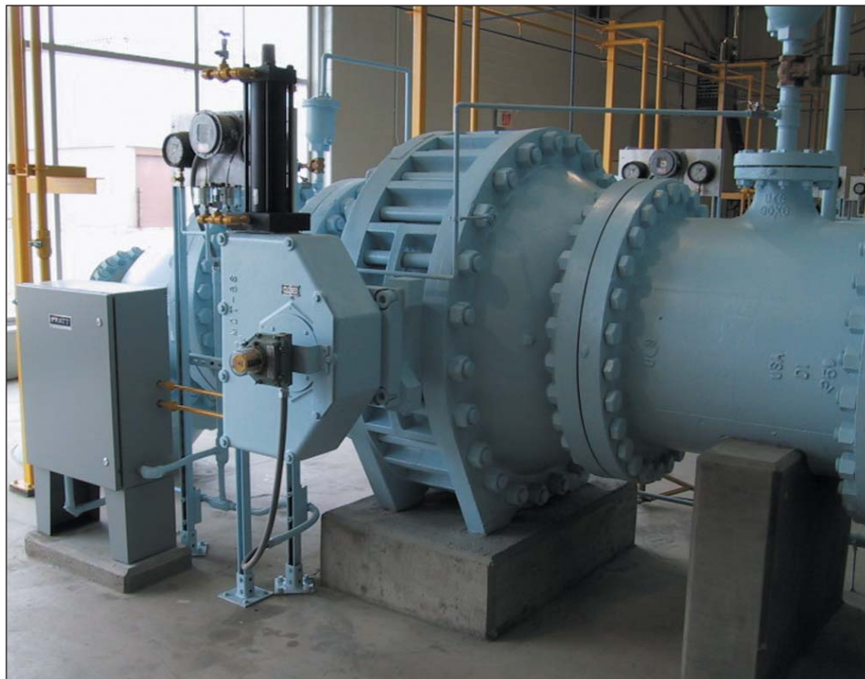
Rubber Seated Ball Valve Installation
